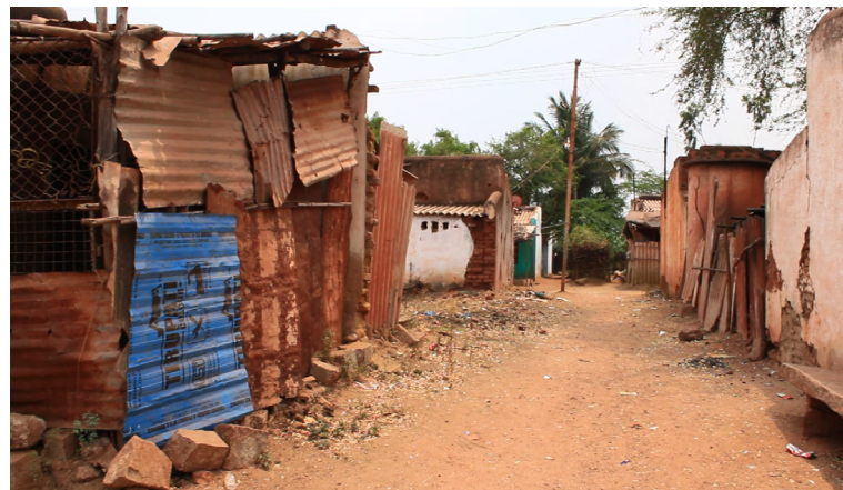
Dilapidated living quarters at the colony
