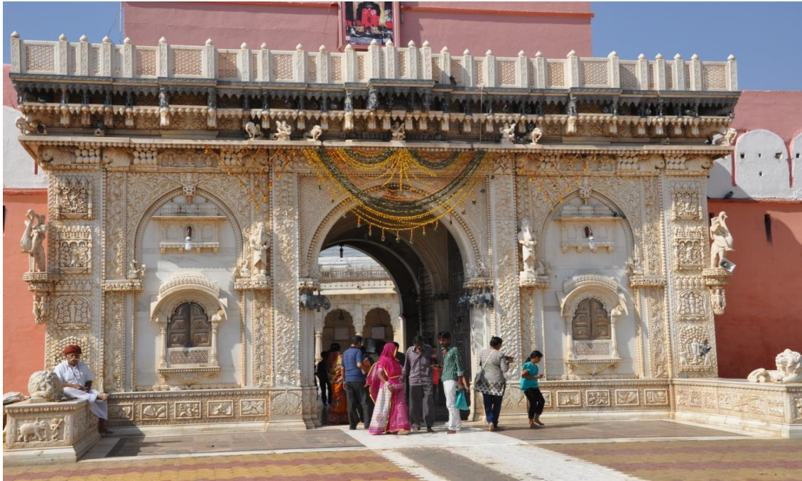
Deshnok Temple in Bikaner district, an example in excellence in marble
